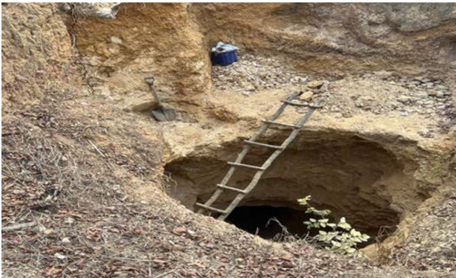
Plate 2. Mining shaft accessed via an improvised wooden ladder, with high instability and safety risks
