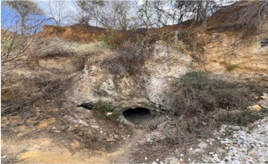
Plate 1. Extraction front on a slope with instability risks, where access is narrow
